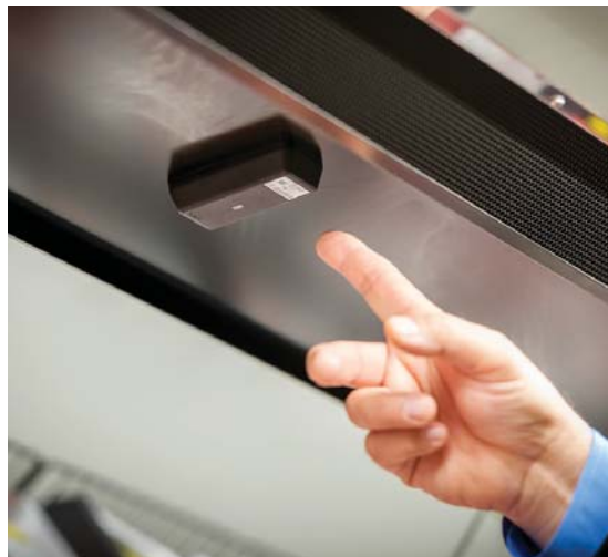
COLD ENOUGH A meat department associate stocks the shelf beneath a temperature-monitoring sensor, which immediately detects any cooling system malfunctions
